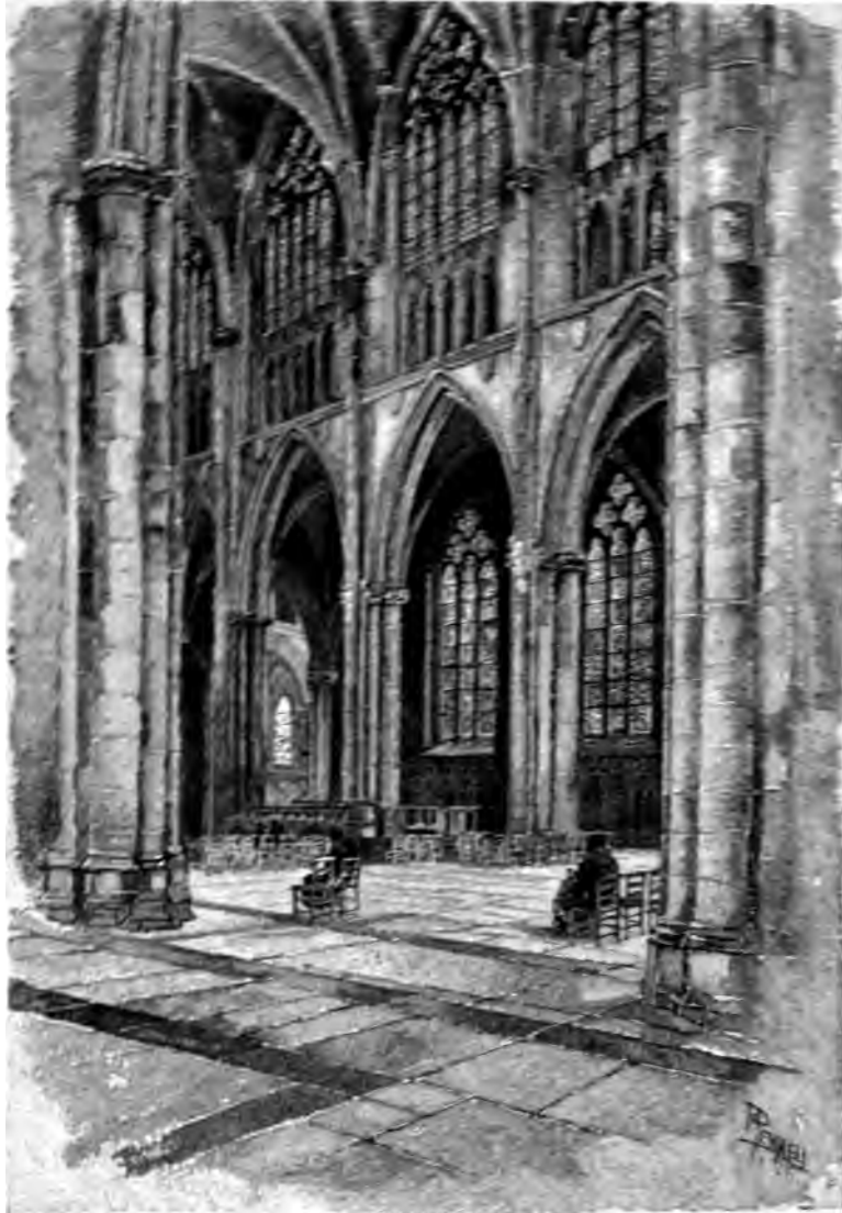
THE NAVE, FROM THE NORTH AISLE.
